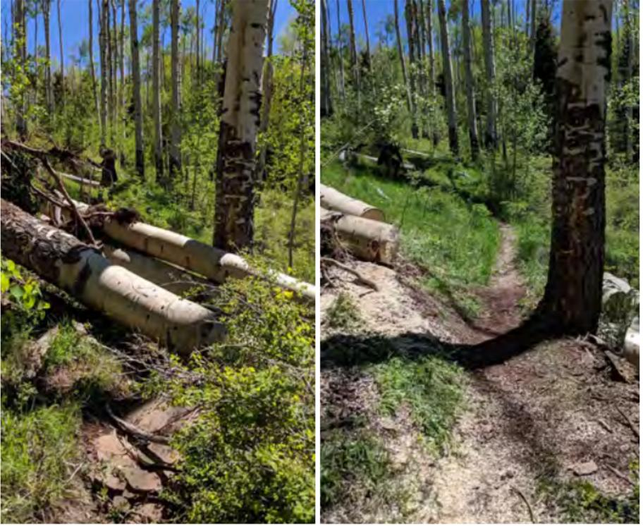
**Figure 3–11.** When logging out a trail on a hillside, make sure to clear the uphill side far enough off the trail in case the log slides down over time. San Juan National Forest, Colorado. USDA photos by Chris Bouton.
