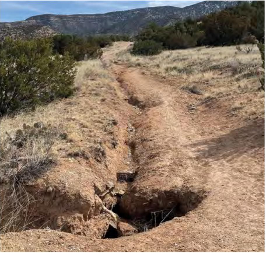
**Figure 2–6.** Water has concentrated along the berm, causing erosion. Cibola National Forest, New Mexico. USDA photo by Kerry Wood.
