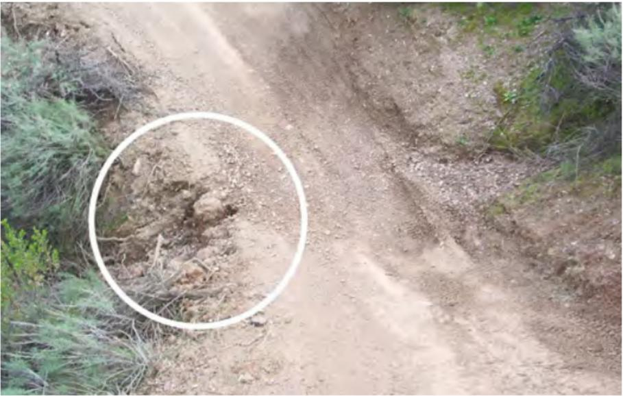
**Figure 3-16.** Headcut starting from water leaving the trail at too high of a velocity and creating a waterfall effect. Los Padres National Forest, California. USDA photo by Scott Johnson.
