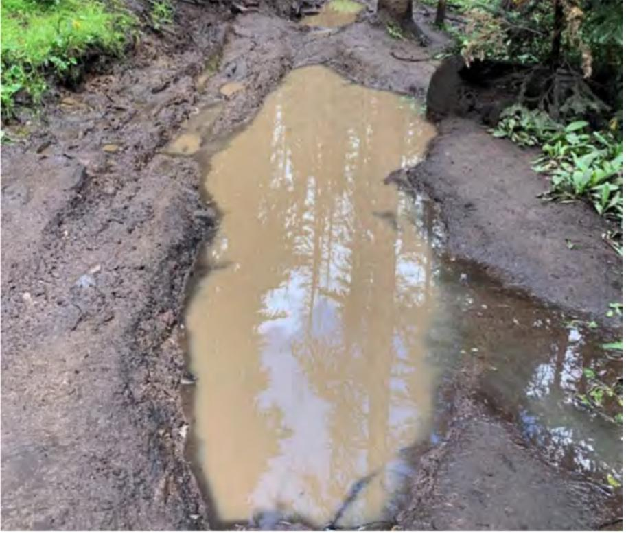
**Figure 4-1.** Water pools in ruts created when the trail is saturated. Solutions for this include more effectively removing water from the trail, installing a forced uphill undulation, or hardening sections where rerouting isn't possible and draining is not effective. USDA photo.
