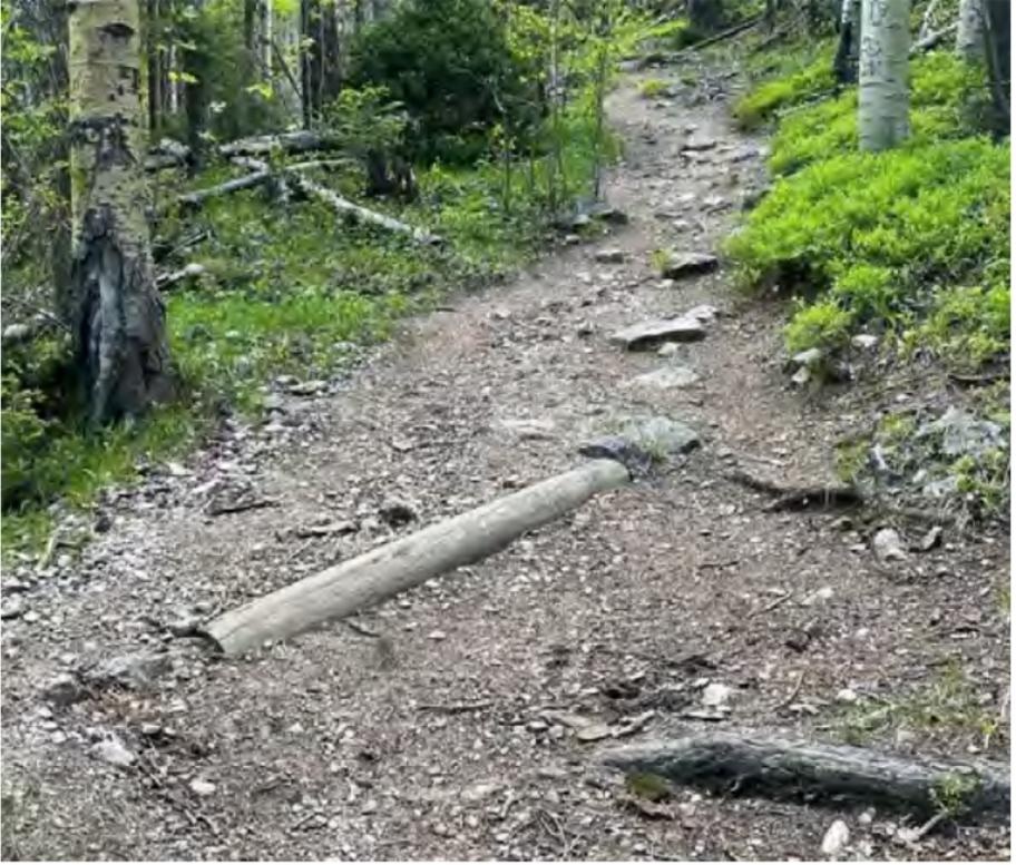
**Figure 4–7.** Waterbars fail for a variety of reasons and are not a preferred way to drain water off the tread. Water and sediment load have overwhelmed this waterbar and users have begun skirting around it. Carson National Forest, New Mexico. USDA photo by Kerry Wood.
