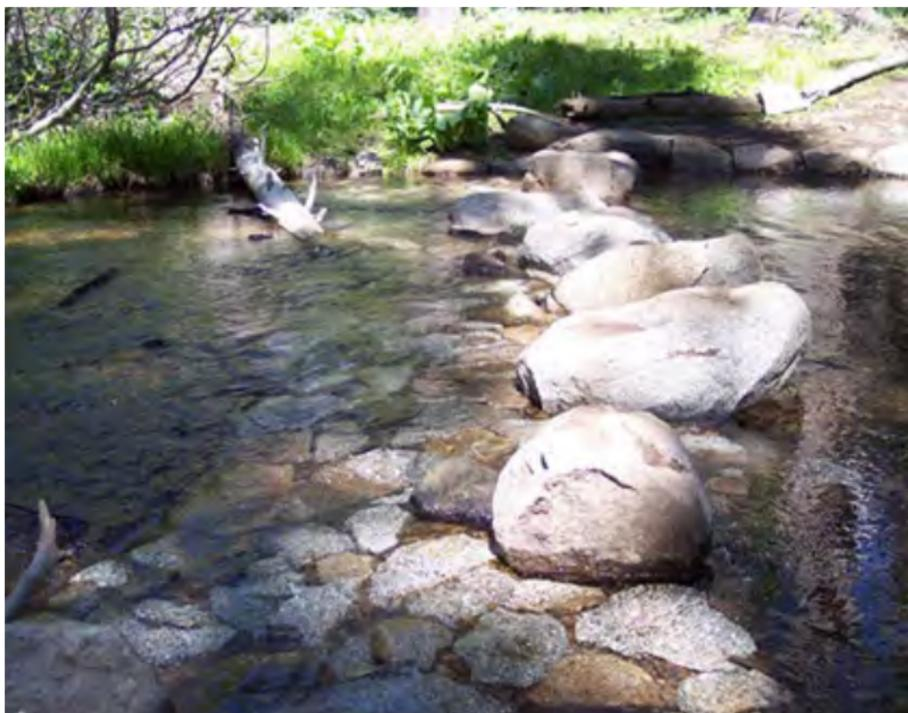
**Figure 4-12.** Fords should be established in wider, shallower portions of a stream. Place steppingstones for hikers. Approaches should climb a short distance above the high-water line. Lake Tahoe Basin Management Unit, California. USDA photo by Garrett Villanueva.
