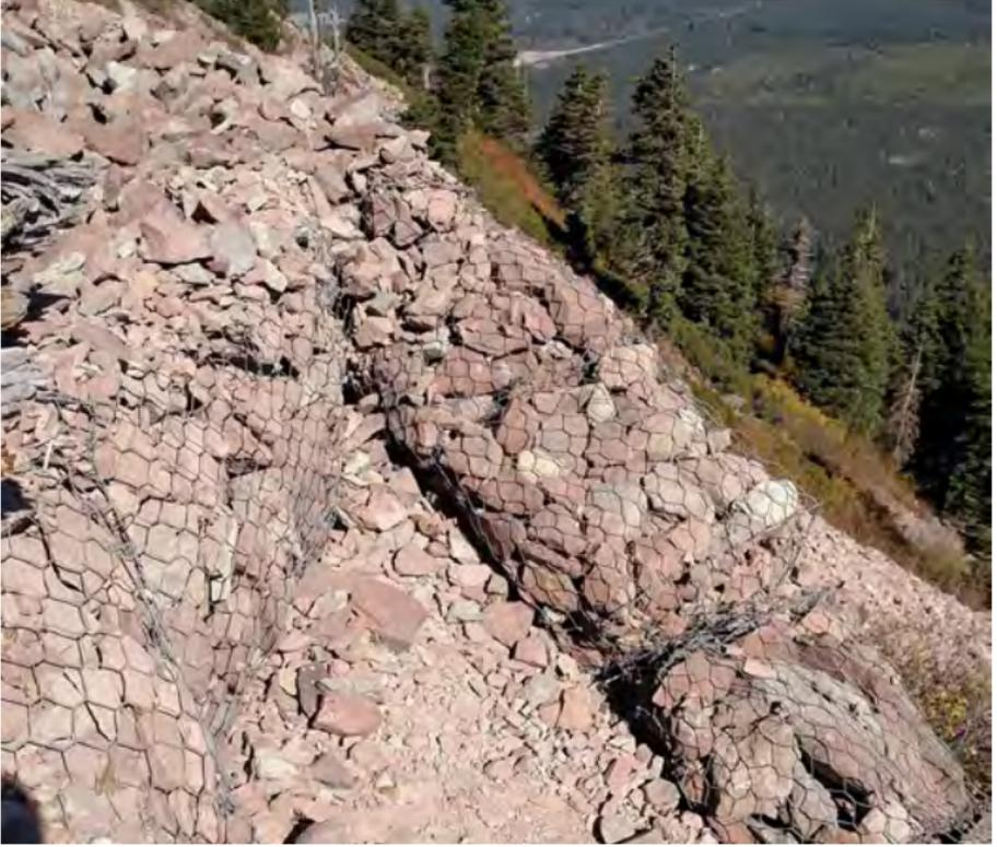
**Figure 4-46.** Place rock tightly to avoid failure. This failing gabion was constructed with inadequately sized material and without sufficient batter. Shasta-Trinity National Forest, California. USDA photo.
