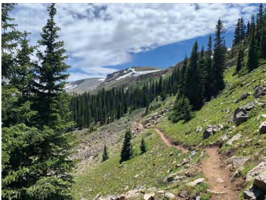
**Figure 2–2.** A physically sustainable trail doesn't depend on building drainage structures to drain water off the tread and resist erosion. It is aligned along the elevation contour with an undulating pattern of crests and dips, called grade reversals. Pike-San Isabel National Forests, Colorado. USDA photo by Dani Cook.
