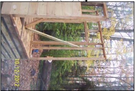
FRONT/BACK WALL BRACING
