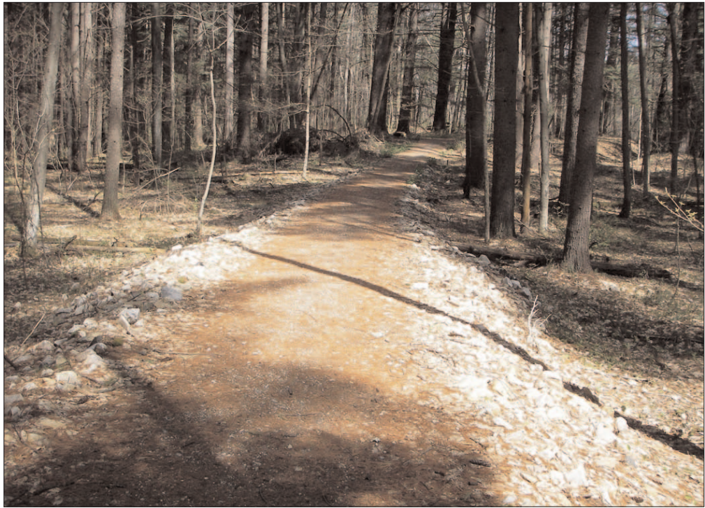
Several short sections of the Falls Village Trail had to be built up with imported rock to meet accessible grade guidelines.
