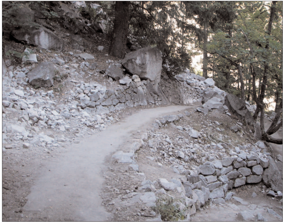
This trail requires cribbing, in this case made of stone, to prevent the backslope from sloughing on to the treadway. This cribbing is typical where bench construction is used on steep slopes.
