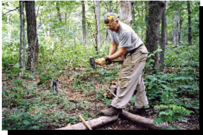
Figure 9. Tent pad logs should be embedded and anchored with rebar or visitors may pull them out for firewood.
