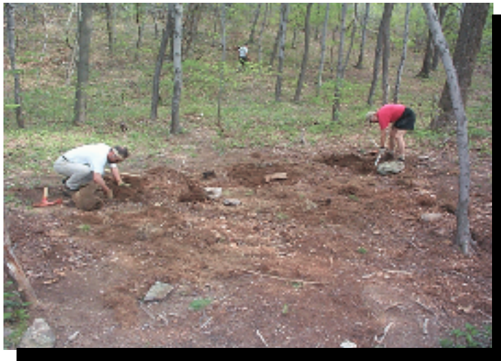
Figure 12. Club members ice-berging rocks to close this tent-site and shift use to adjacent constructed tent-pads near Maupin Field shelter, Virginia.
