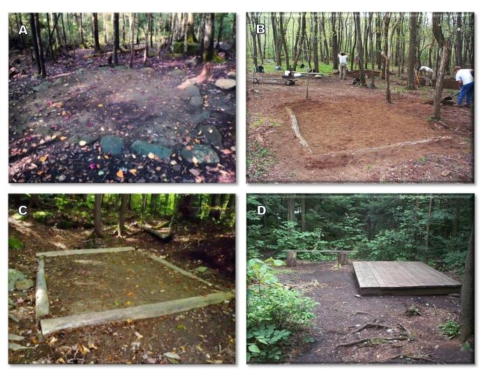
Figure 13. A) Rock-lined tent pad, B) Embedded logs pinned with rebar, C) Wood-lined tent pad, and D) Wood-decked tent platform.
